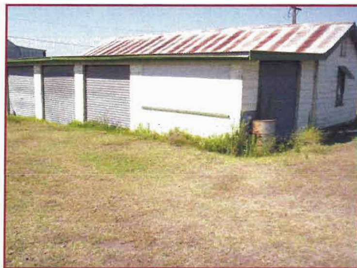
Photo 18 – Former dairy shed, looking south-east.
