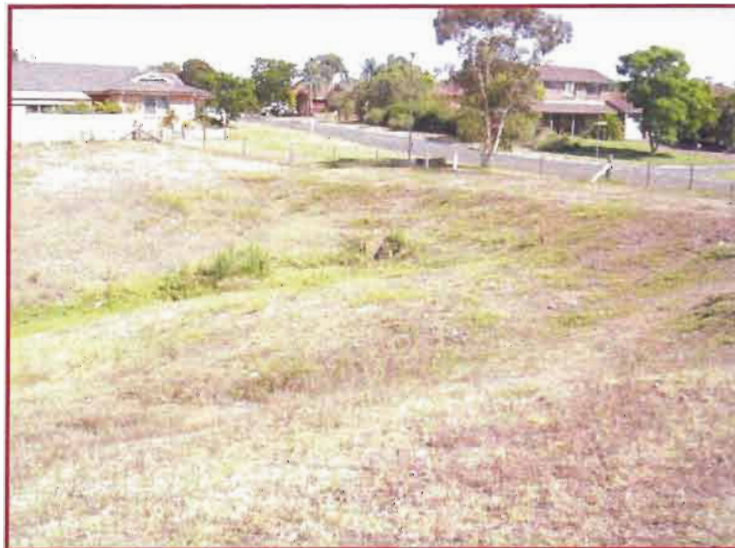
Photo 5 – Stormwater culvert draining onto site looking north-west
