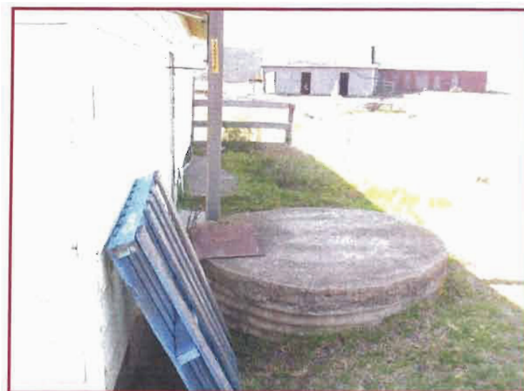
Photo 21 – Stormwater collection tank next to the dairy shed. Looking east toward the storage shed.
