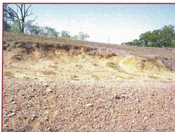
Photo 10 – Erosion scarring along the gully banks
