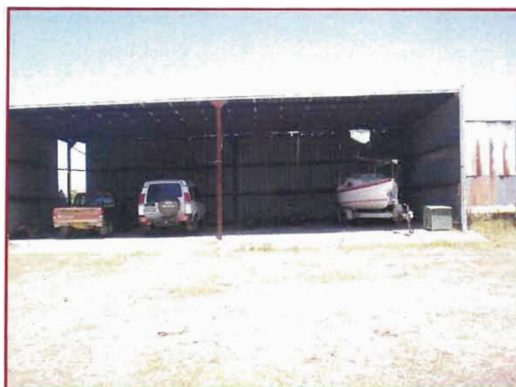
Photo 19 – vehicle storage shed, looking south.
