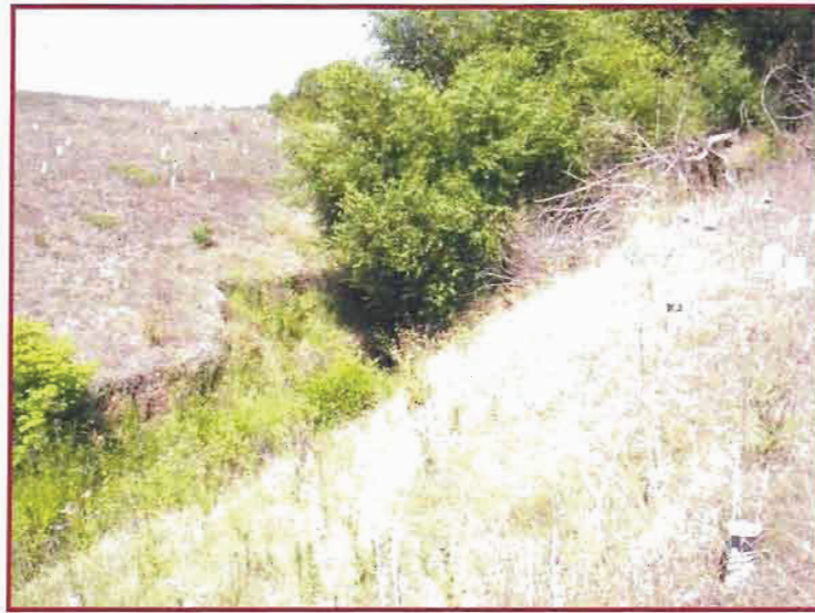
Photo 2 – Typical section of the gully, looking west. Some erosion scarring is visible along the southern side of the gully.
